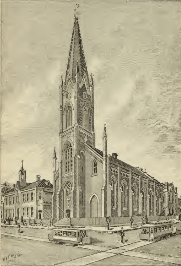
ST. MARY'S CATHOLIC SCHOOL AND CHURCH.
